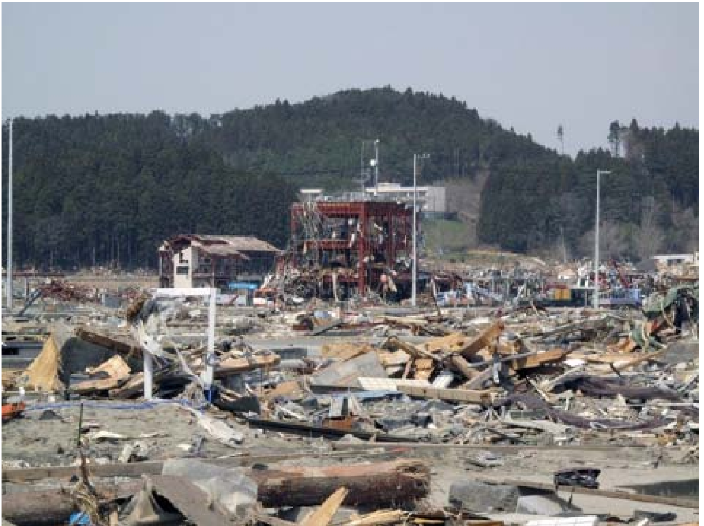
Disaster Prevention Center. Photo by Koichi Hasegawa.
