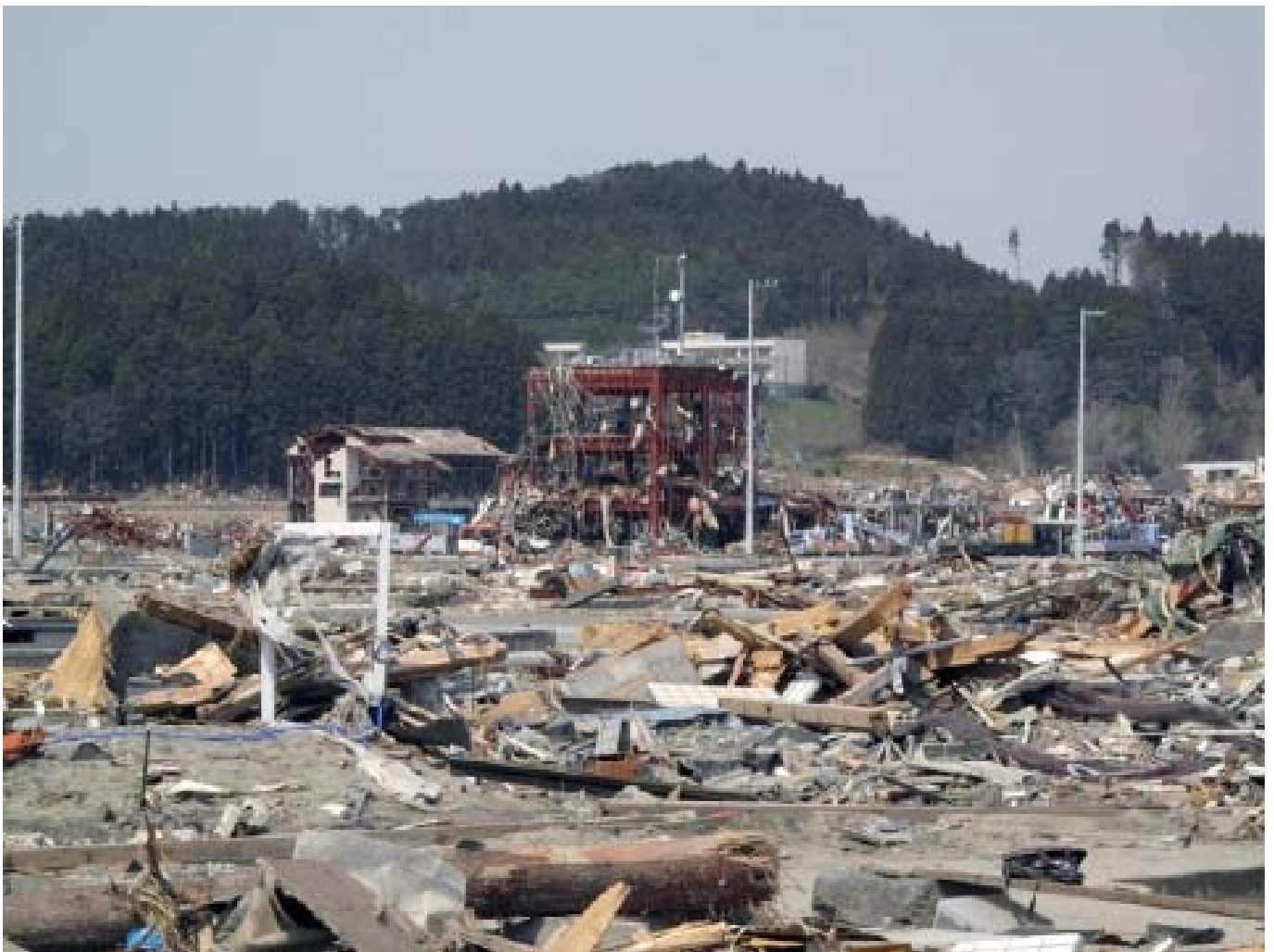
Disaster Prevention Center. Photo by Koichi Hasegawa.
